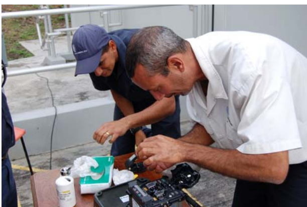
Staff splicing external fibre to internal fibre.
