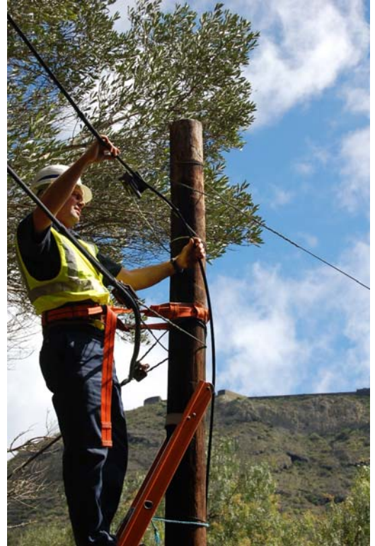
Service Provisioning Staff securing external Fibre cable along aerial route.
